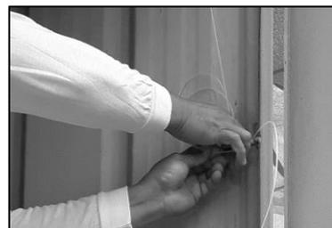
8.11.2. Pull the rope out of the container to provide space between the roof and liner for air circulation.
