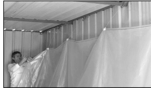
8.3.8. Apply proper tension and secure the nylon rope to minimize the sagging of liner for ease of loading.
