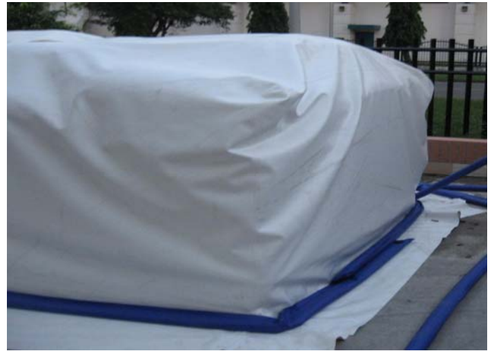
Water snakes placed along the perimeter
