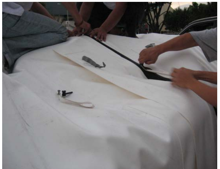
Zipping of left, middle and right cover section
