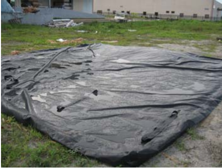
Fully covered and protected during rain
