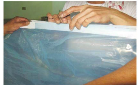
Sealing of liner using gas tight tape
